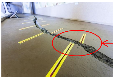
Figure 1 The “Faulted Floor” in the Fremont Community Centre, California caused by the Hayward Fault ( Source: Mercury News Archive)
