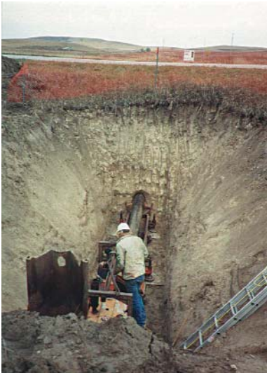
Workers prepare to install a water main under a highway by boring and jacking.
