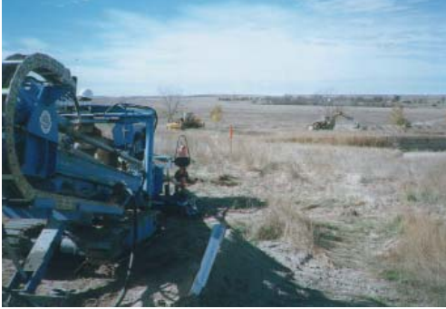
Directional drilling takes place under the White River for service line installation on the United States largest rural water project.
