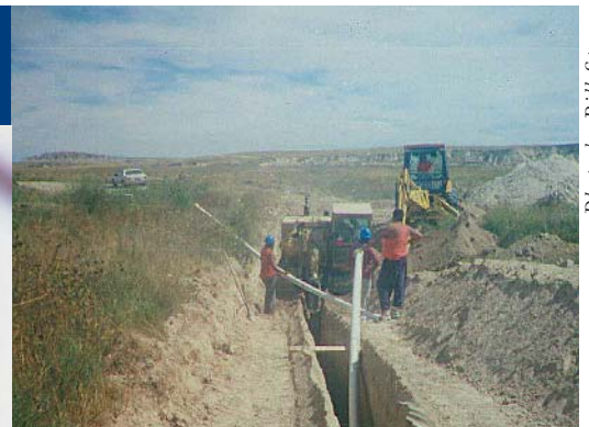
Workers on the Mni Wiconi project are trenching and installing pipe for water distribution on the Pine Ridge Reservation.
