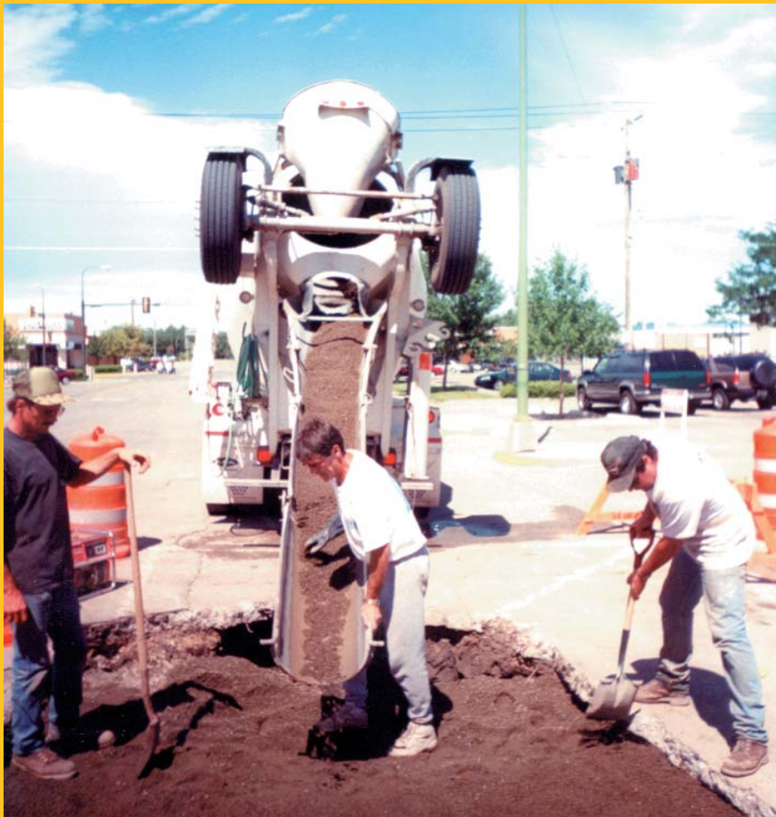
City of Rapid City employee and Terry Collins (center) pour the glass and concrete mixture into its first pavement patch.
